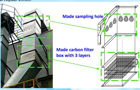
SRV has renovated the carbon filter cartridge and renewed the sampling pit in some exhaust gas treatment systems to increase the efficiency of odor and organic vapor treatment.
